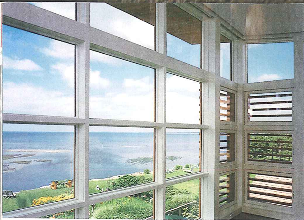
IN A MARRIAGE OF FUNCTION AND BEAUTY, THE TAYLOR HOUSE FEATURES HORIZONTAL CYPRESS LOUVERS THAT PERMIT YOU TO SEE OUT WHILE RETAINING PRIVACY FROM THE OUTSIDE.
